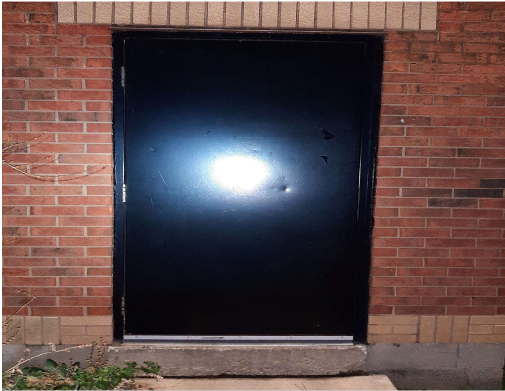
Photograph No. 1 – Exterior black paint is lead-based.
