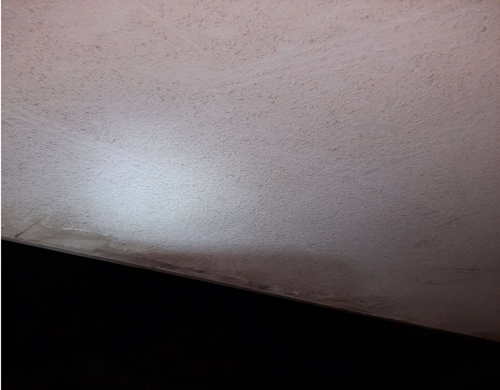
Photograph No. 5 – Texture coat on exterior overhang is non-asbestos.
