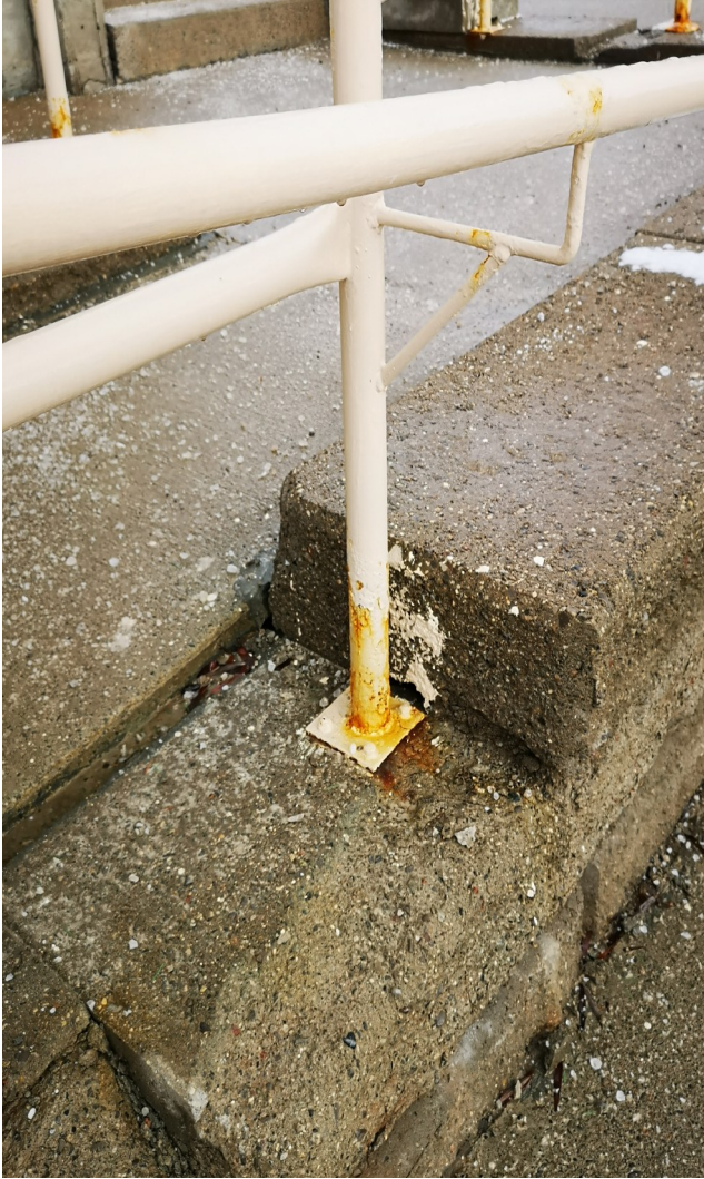
Fig. # 5 Deteriorated ramp and side retaining stones. Fig. # 6 Deteriorated side retaining stones. Note stone are uneven.
