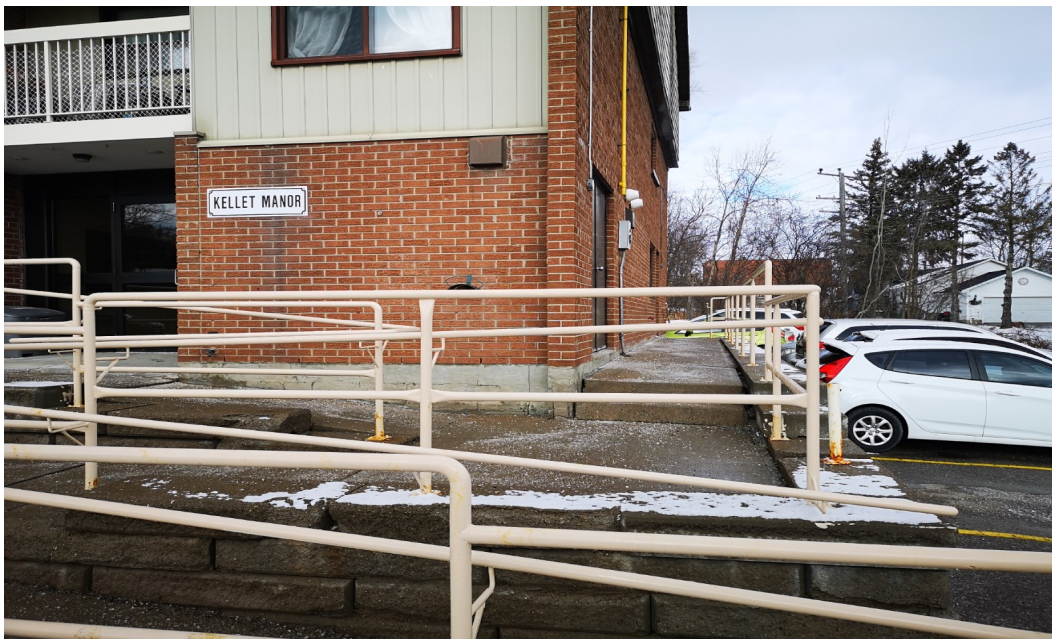
Fig. #2 General view of main entrance bottom part of the ramp.
