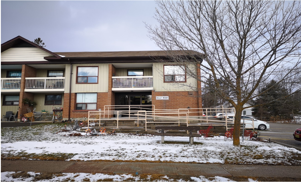
Fig. #1 General view of main entrance ramp.
