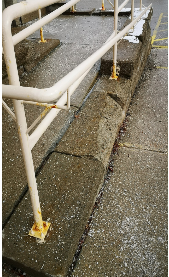
Fig. # 5 Deteriorated ramp and side retaining stones. Fig. # 6 Deteriorated side retaining stones. Note stone are uneven.
